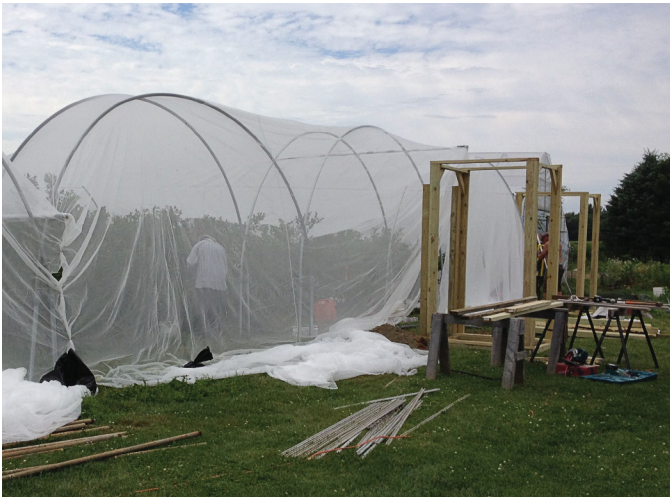
Installing exclusion netting over hoops previously used for a high tunnel to protect blueberries. The 0.95 mm × 0.95 mm (80 gram weight) insect netting prevents SWD from gaining entry to the high tunnel. Care must be taken to prevent gaps and to exclude SWD when entering and exiting the high tunnel. The wooden frame will be used for a netted double entryway. Photo by Laura McDermott, Cornell University.
